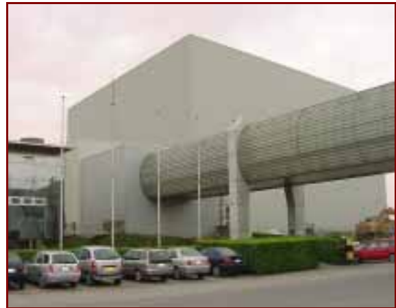
Conveyor Bridge from Production (right) to ACCESS (left)
