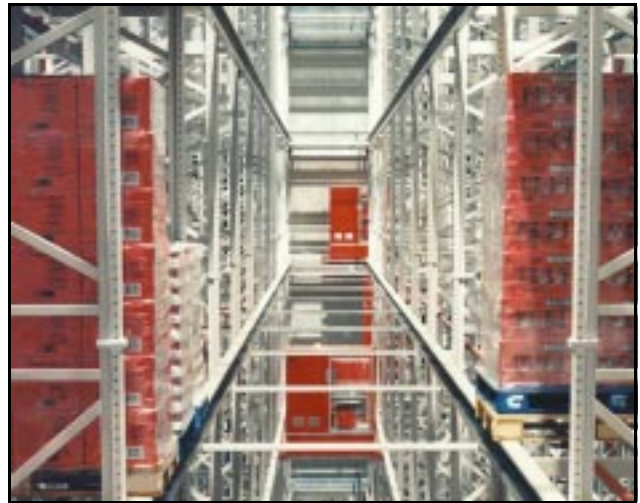
Automated Vehicle in Racking
